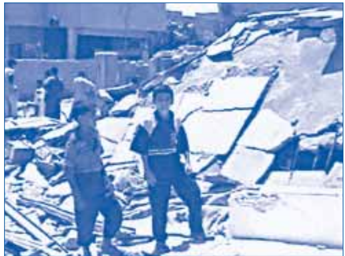
Not-so-safe Safe-house demolished
