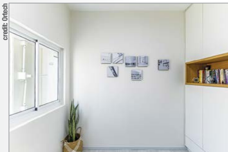
A room whose walls have been reinforced with Ortech's solution
