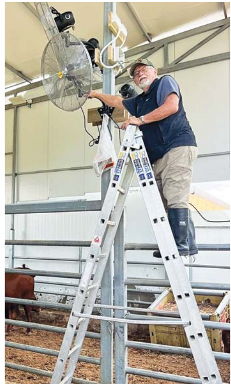
Larry Borntrager installs fans in the calves' shed to protect against the fierce summer heat.
